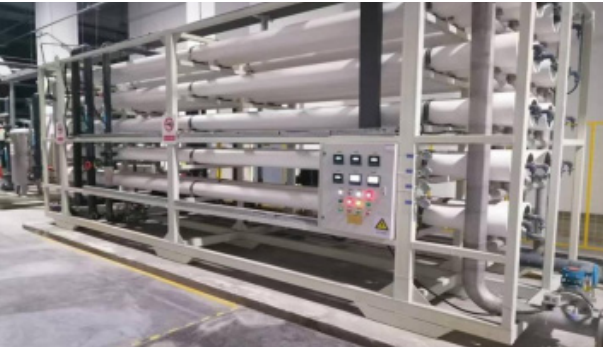
Water Recovery from PW Particle Wastewater Replacement System at Ningxia Zhonghuan
